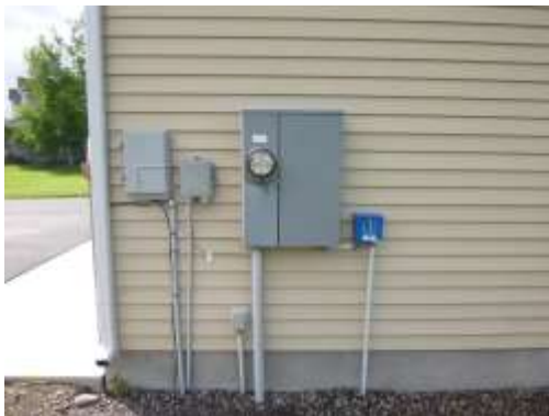
Main Service Entrance
